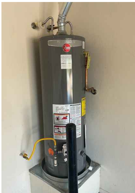
New water heater installed on drain pan
